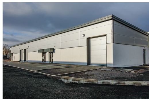
Completed units at Flemington Road, Queensway Industrial Estate, Glenrothes
